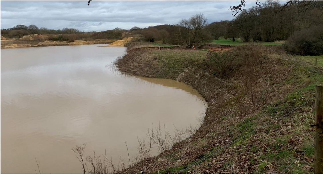
Figure 3: February 2020 – flooded extraction area with river breach top centre, looking east.
